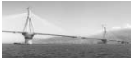
Just a few meters remaining to join the deck.
