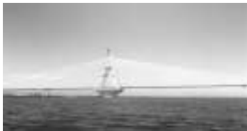
One of the pylons.
