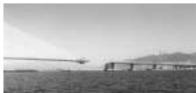
The deck is ready to join the Rio side.
